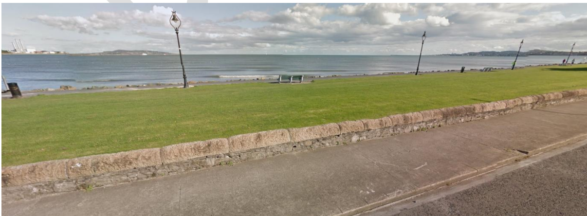
Figure 2.1 – Wall at back of footpath
